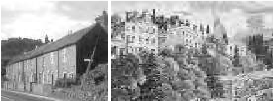
Far Left: Coalbrookdale, Carpenters' Row, cottages built by the company for workers in 1783.
