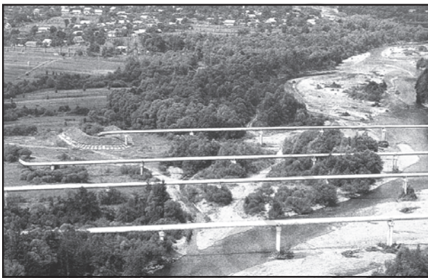
Fig. 7.17: Pipelines transporting natural gas in Ukraine
