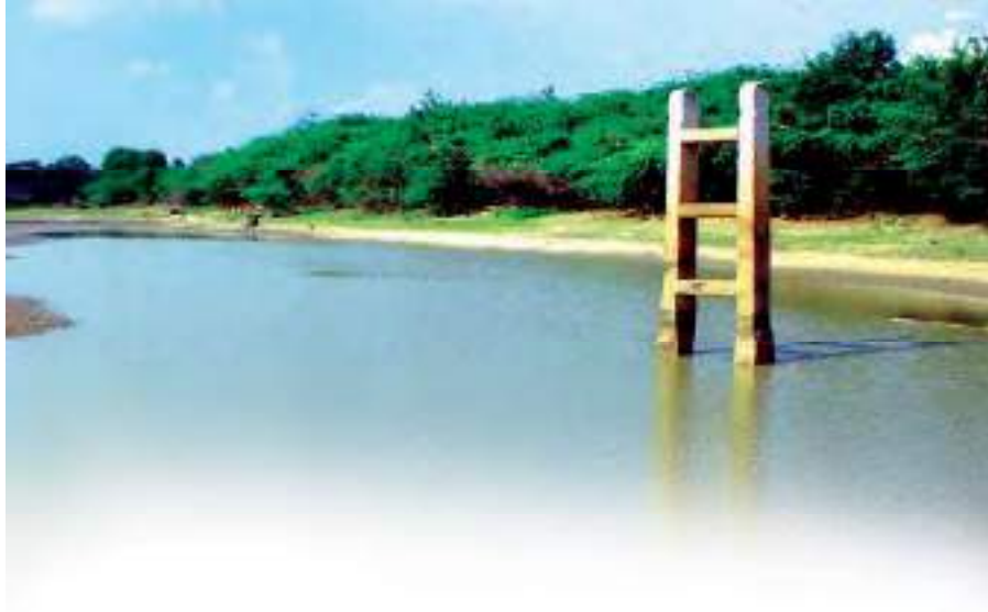
Fig. 5 A ninth-century sluice gate in Tamil Nadu. It regulated the outflow of water from a tank into the channels that irrigated the fields. A sluice gate is traditionally a wood or metal barrier which is commonly used to control water levels and flow rates in rivers and canals.
