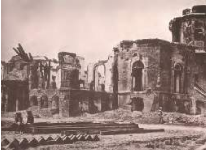
Fig. 17 – Ruins of the Residency in Lucknow
