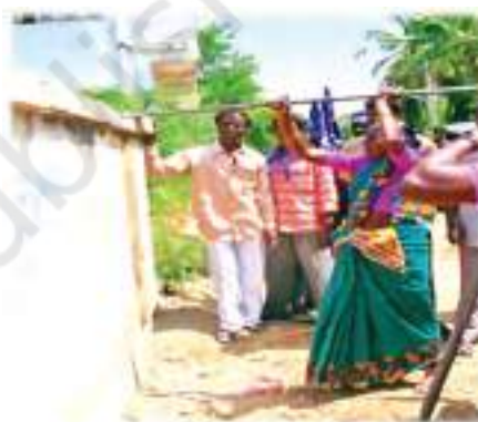
Members of the Safai Karamchhari Andolan demolishing a dry latrine.
